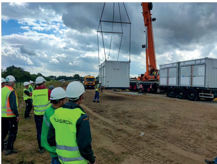
Truck unloading of Sungrow inverters on-site
